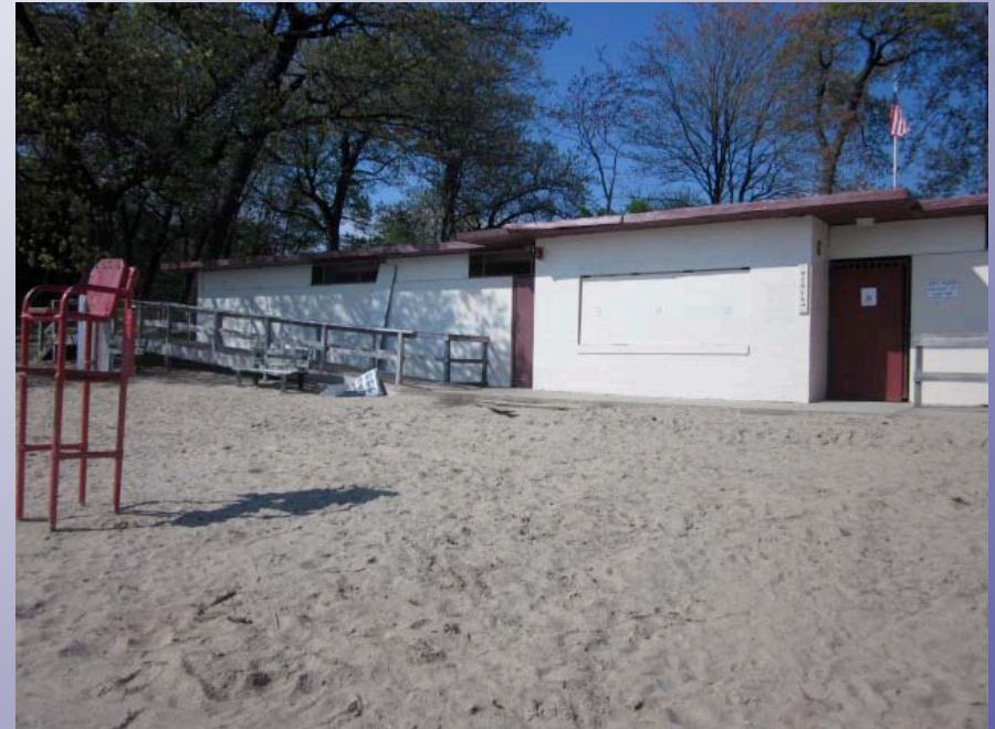
Bathroom & Changing Room Facilities
